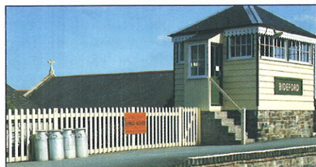
The renovated signal box
